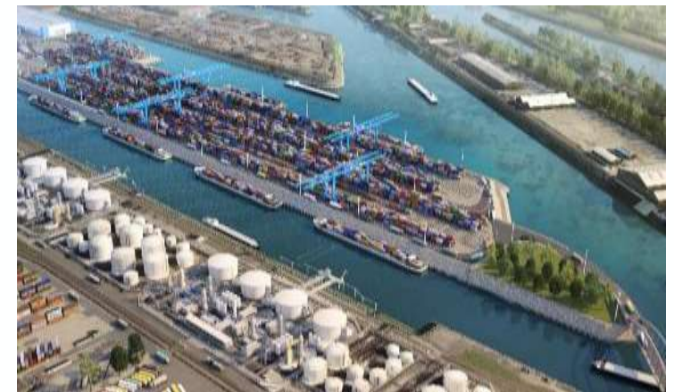
(as of 2022) Duisburg Gateway Terminal
