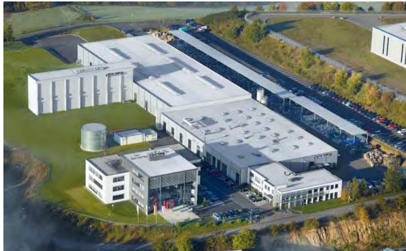
TSUBAKI KABELSCHLEPP Headquarters Wenden, Germany
