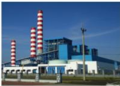
Gas Power Plants
