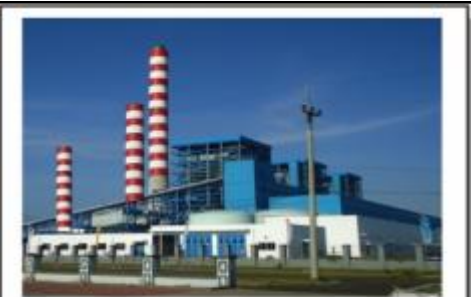
Gas Power Plant
