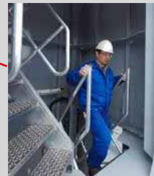
Stairs inside the tower for weather-proof ascent
