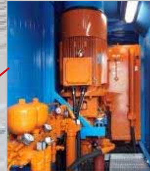
Hydraulics room with main pump and tank
