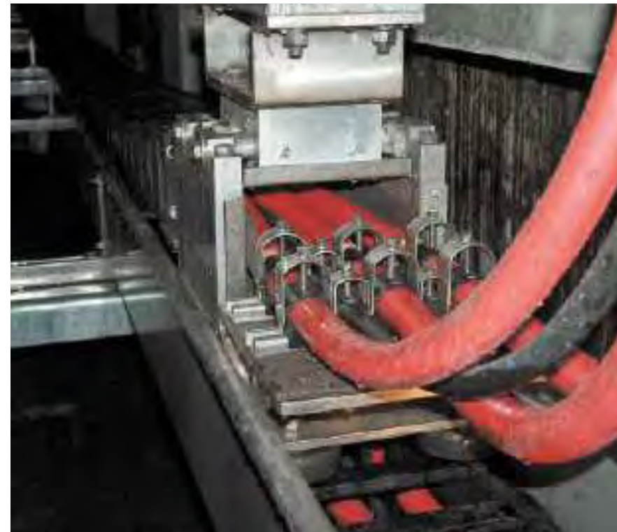
Clamps for safe cable strain relief
