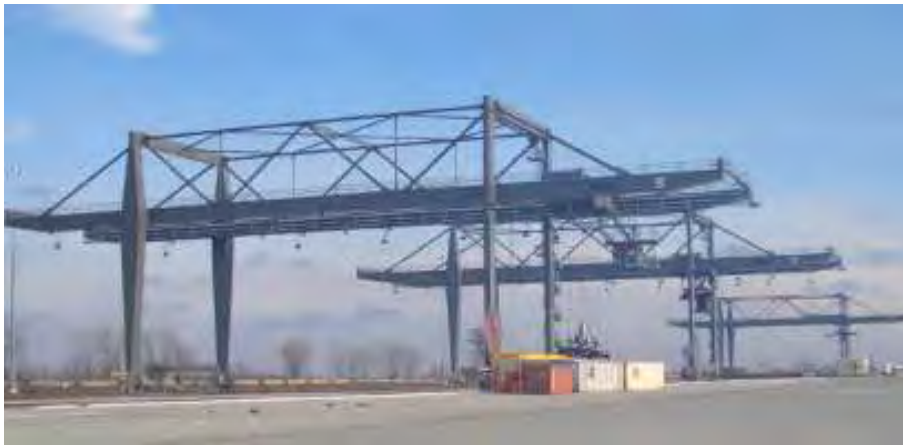
P4.56R-System is running successfully on 5 Künz RMG's
