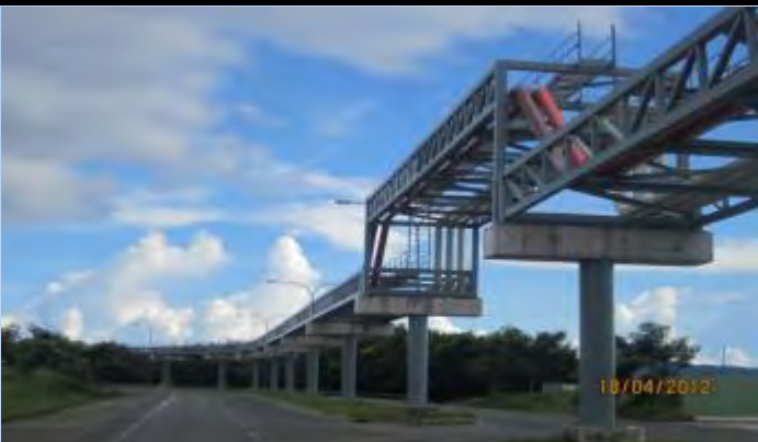
Cargo lines on pipe rack
