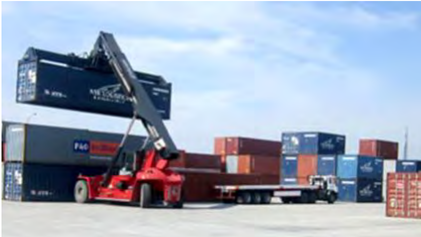
Container Yard: Capacity 400,000 TEUs per annum
