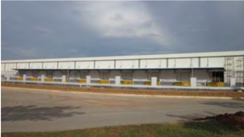
General Warehouse (on progress)
