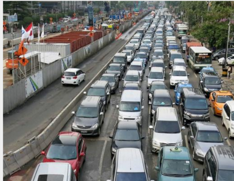
Cars are held up in a traffic jam on a main street in Jakarta on Wednesday while construction of Indonesia's subway is underway on the left.
