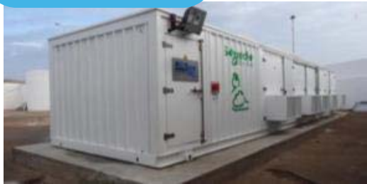
2x2MVA ShoreBoX Navv ships
