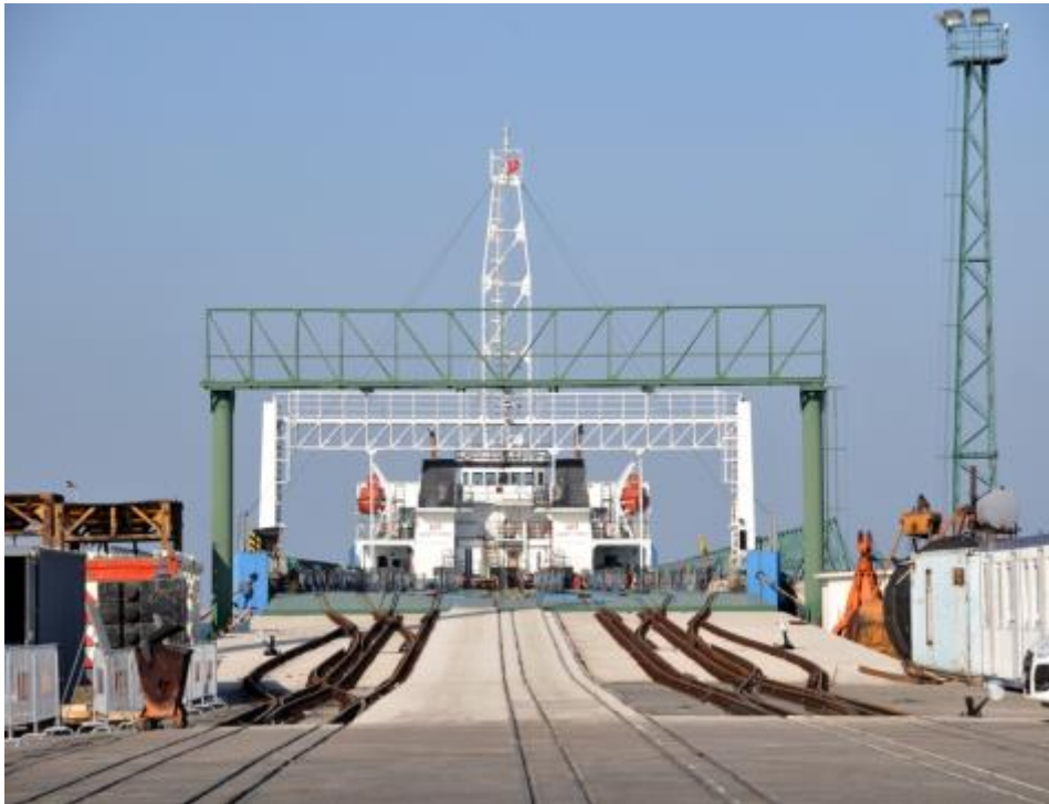
Adjustable rail-ferry ramps (European&Russian Railway System)
