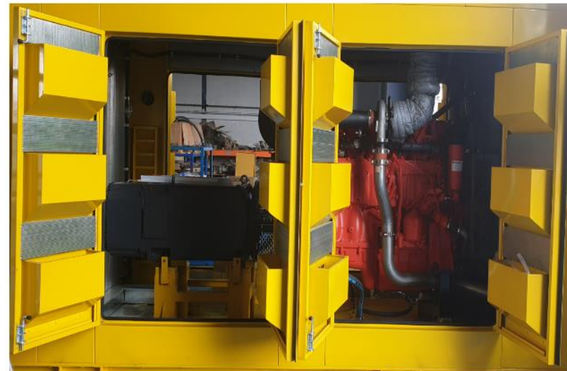
CLEAN PIPING OF EXHAUST INSIDE THE ENCLOSURE
