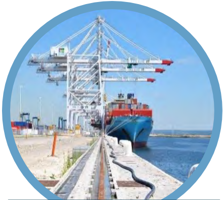
STS Crane Runways and Trolley
