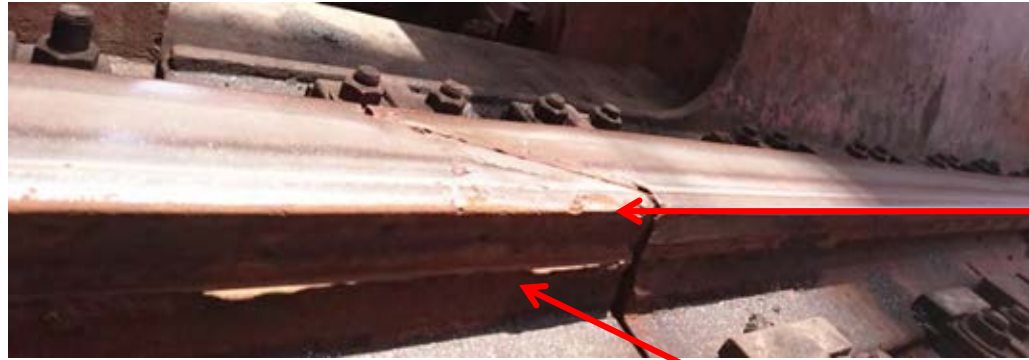
Stiffener Cracks
