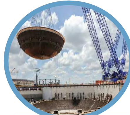
Super Heavy Cranes
