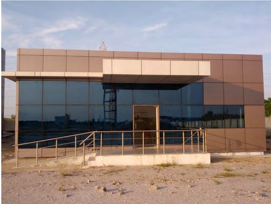
→ CHAs Utility Building
