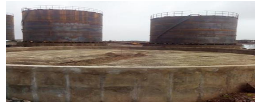
Tanks under construction
