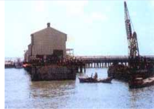
Tata Power Company Limited- Caisson & piled jetty for Trombay units 5 & 6
