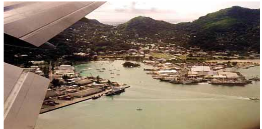
Republic of Seychelles Ship repairs complex -Port Victoria
