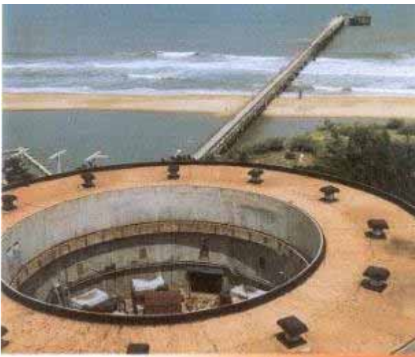
Madras Atomic Power Project Intake structure and submarine tunnel at Kalpakkam
