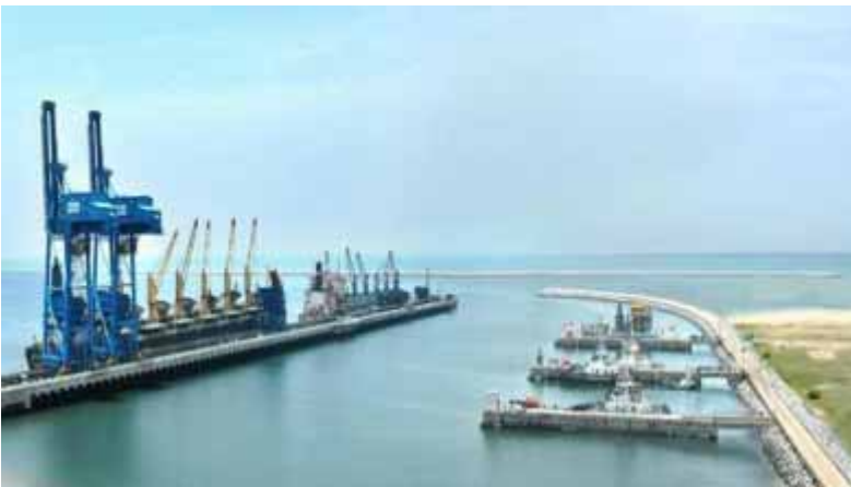
Ennore Port Limited - Capital dredging phase II
