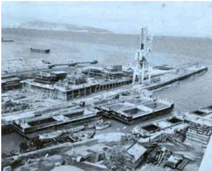
Mazagon Dock Limited- Repairs and rehabilitation of slipway
