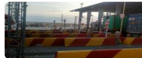
Upgrading the gate complex and systems
