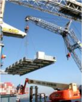
Rotterdam, the Netherlands Upgrade of 12 non-Kalmar STS cranes ▪ 8-metre height increase ▪ 4-metre boom extension ▪ Stacker platform ▪ Lifetime extension
