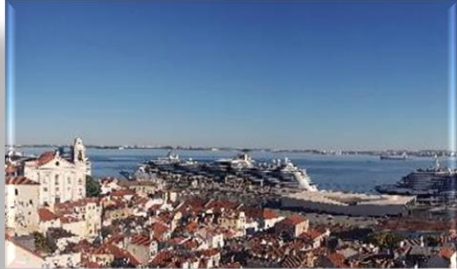
On Shore Power Project: Cruise Terminal and Eastern Zone Terminals
